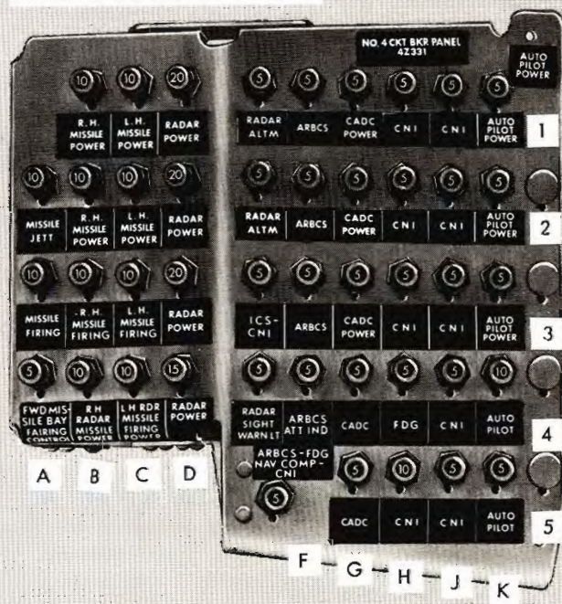
CIRCUIT BREAKER PANEL NO. 4
